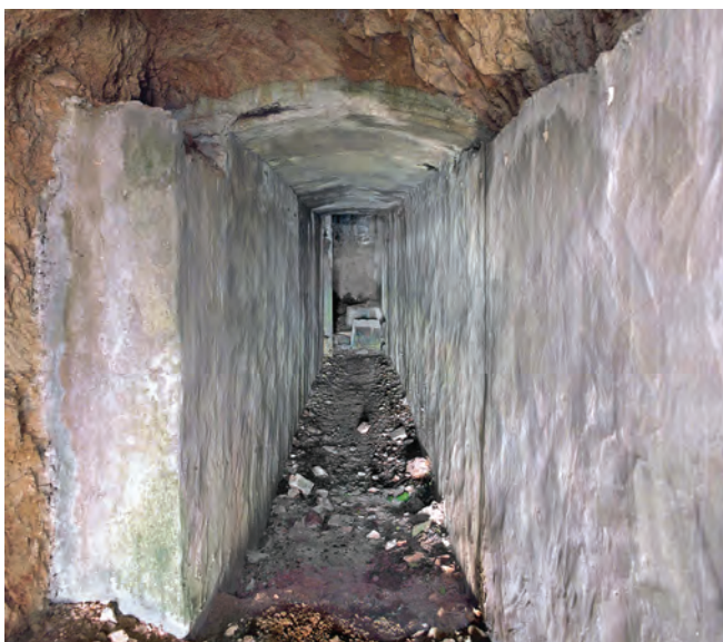
At Lager Sylt the access to the Camp Commandant's house, which was outside the main compound overlooking the sea, was through this short tunnel from the washroom and coal store.
